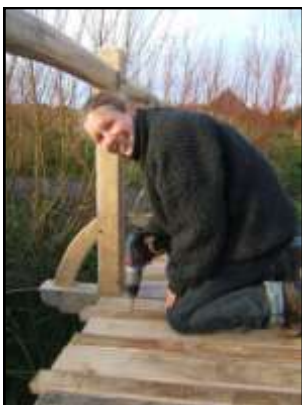
Volunteer working on the new bridge
